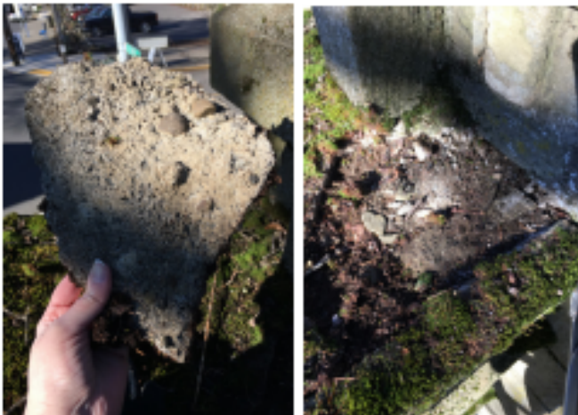
Condition of concrete topping on SE 32nd/E Burnside arch beam.
